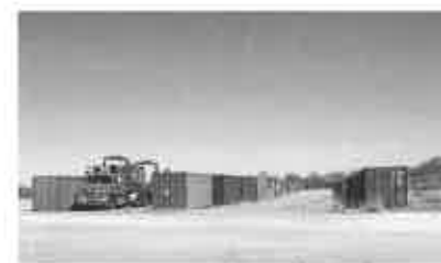
3. Unloading 17 Construction Squadron Containers at RAAF Base Curtin. The container line.
