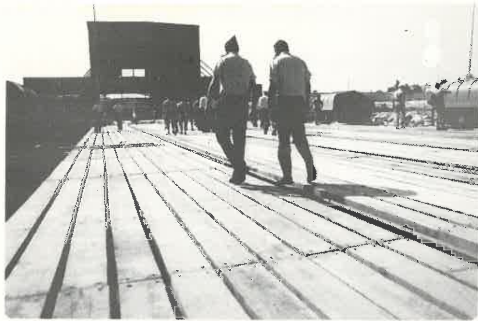
New patrol boat facility at Darwin.
