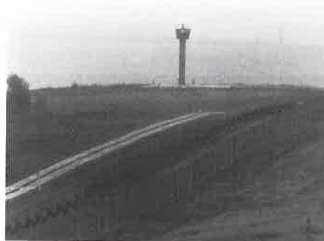
Observation tower near Helstedt autobahn checkpoint
