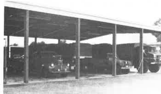
Centre Bay with workshop area on the left.
