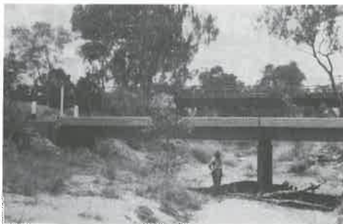
Low level road and high level railway bridge.
